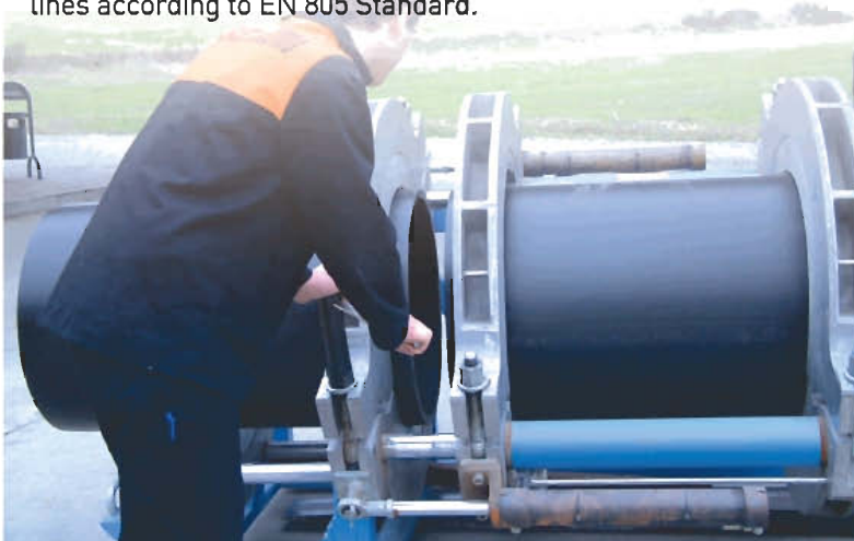
FKS pipe butt welding joint point section.
