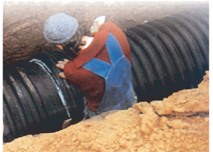
Socket-Gasket section of FKS pipes picture.
