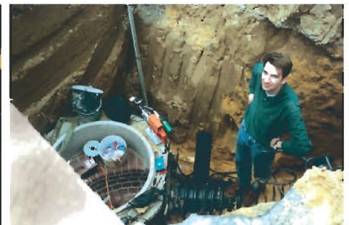
Concrete manhole application
